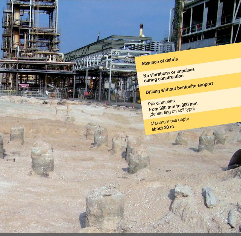
If soil removal has to be minimized during foundation works, displacement piles can be the solution.
