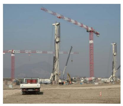
For the construction of Discrepiles, the jobsite has to include a **drilling rig**, a small-sized **tracked hydraulic pump**, a **backhoe excavator** for debris handling and an **auxiliary crane** for cage positioning, if needed.
