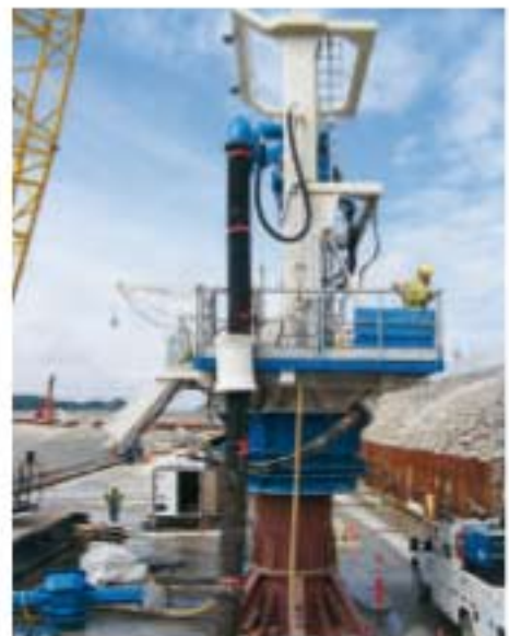
Installation of secant piles in technical area #1
