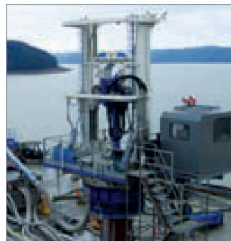
Piling for the dam
