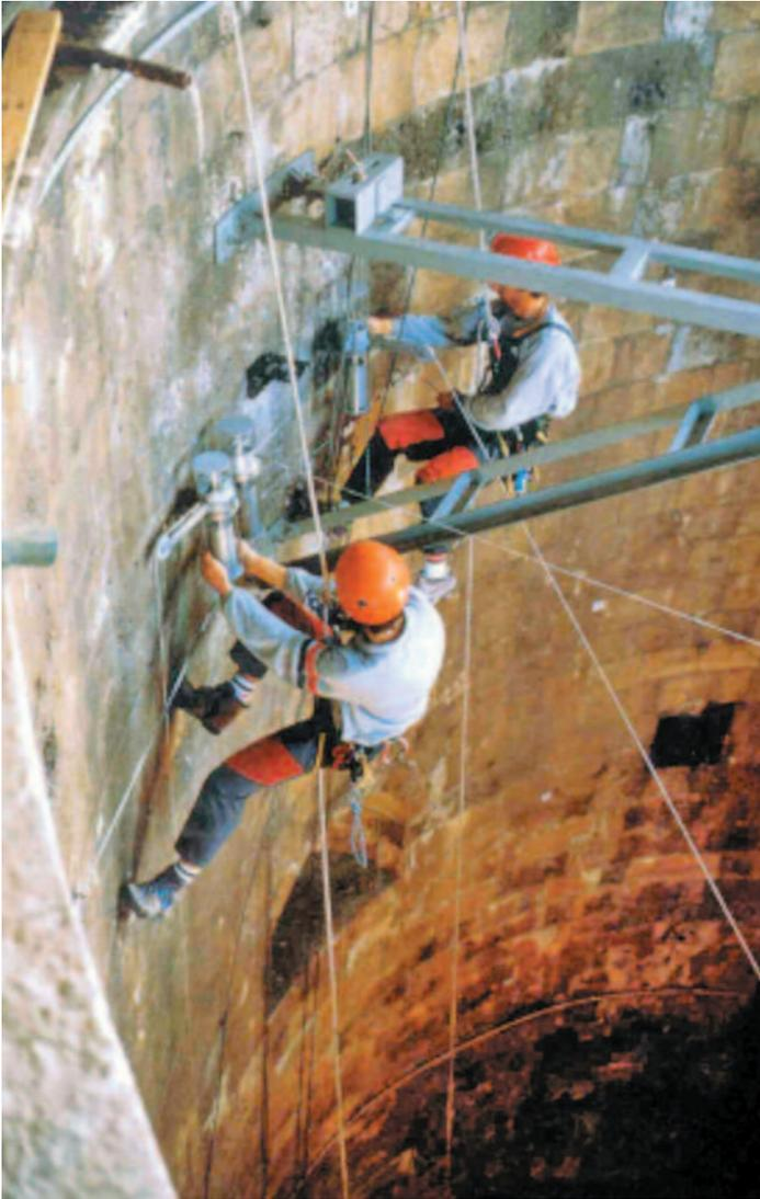
*Installation of complex monitoring equipment to allow continuous measurement of the Tower's displacements, rotations, stresses, temperatures and vibrations.*
