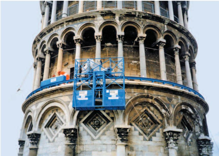
*Steel cables sheathed in Teflon being positioned and tensioned around the first story cornice with a specially-designed device.*
