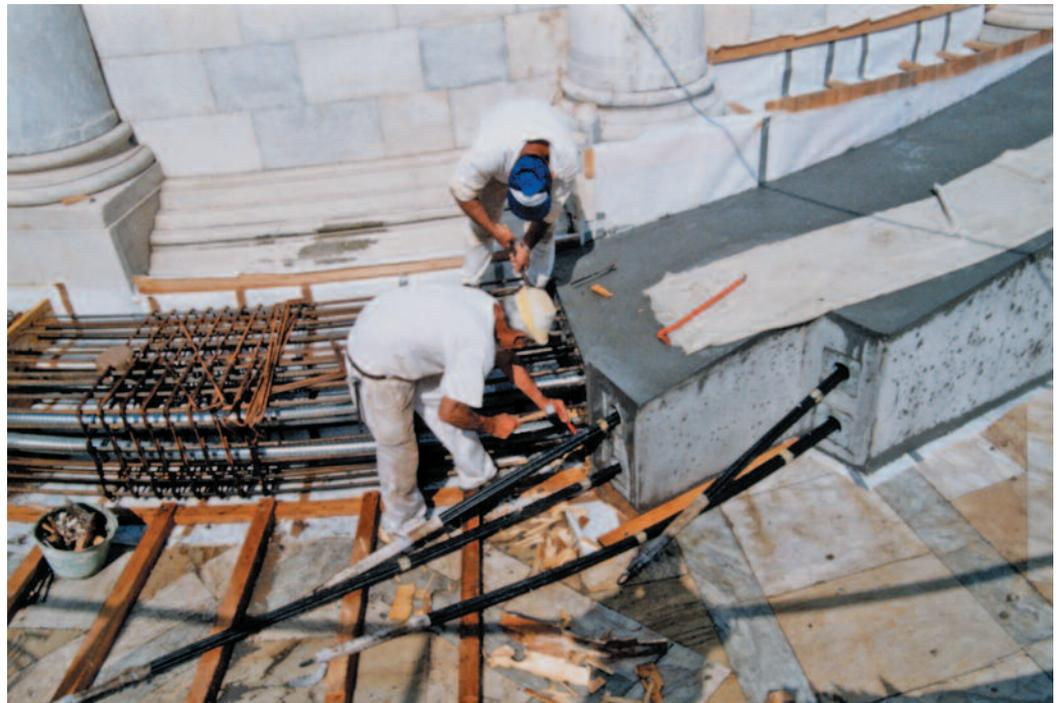
*Construction of the removable concrete ring around the Tower foundation.*
