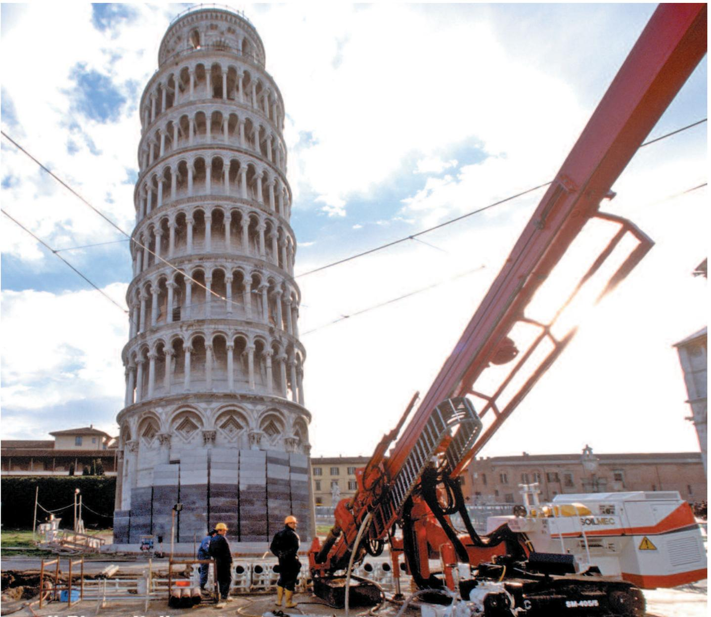
*The temporary post-tension concrete ring with lead blocks stacked on the north side of the Tower foundation. The backstay cables are also visible.*
