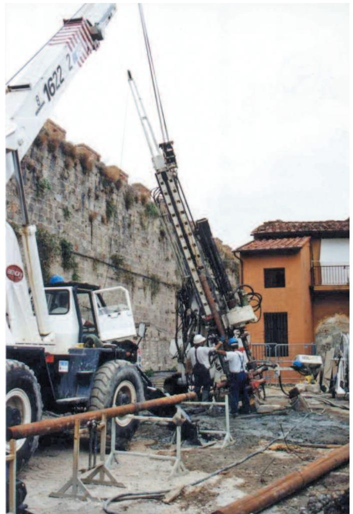
*Temporary rigging trestle used to attach a backstay to the Tower, to prevent potential movement of the Tower during restoration operations.*
