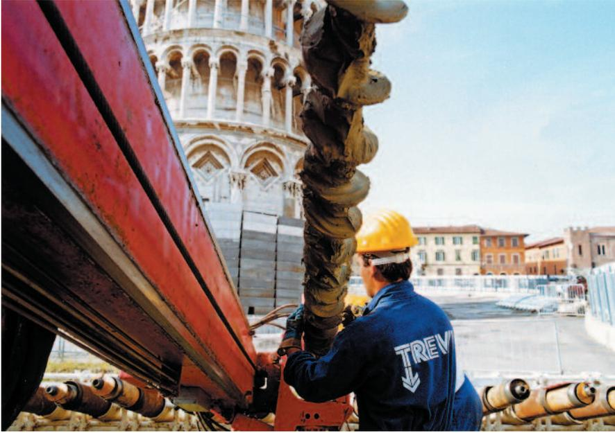
Soil excavation from under the Tower during the final geotechnical stabilisation.
